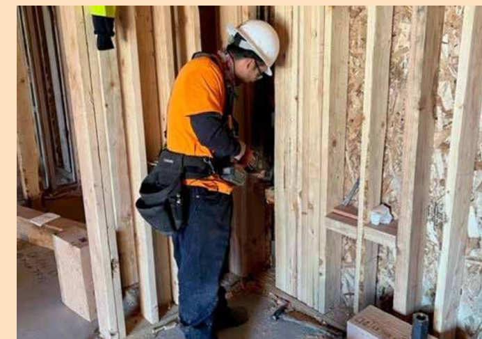
PVJOBS participant Victor Henriquez shown working at an assigned construction project.
