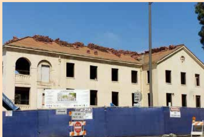
Building 207 under construction at the U.S. Vets development project in Westwood.
